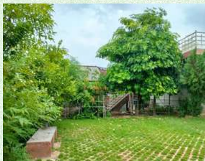
Permeable grass pavers in Chitrawad, Gujarat, support groundwater recharge and reduce flood risk
