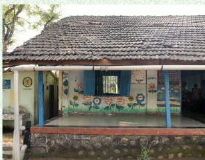
Rooftop rainwater harvesting structures enhance groundwater recharge, helping replenish local aquifers
