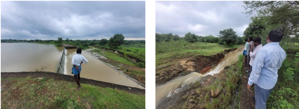
Figure 14: Desilted pond to mitigate annual flooding and increase storage in Ainapur Village
