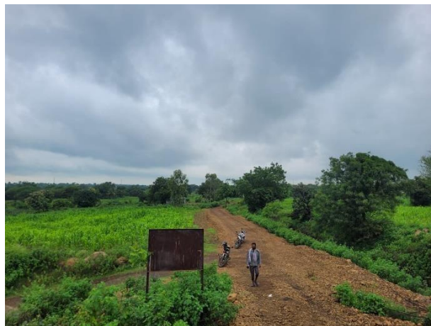
Figure 15: Silt from desilting of the pond repurposed to construct roads in Ainapur Village
