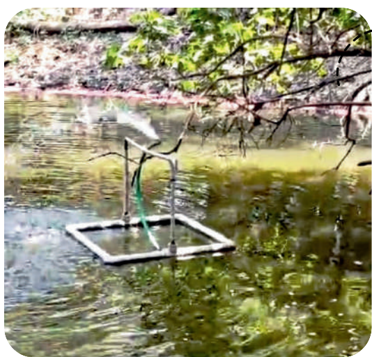
Solar Powered Filtration System
