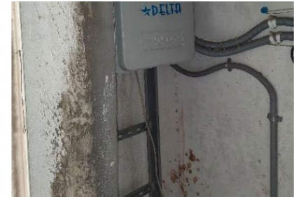
Box for aggregator for overdeck sensor data logging
