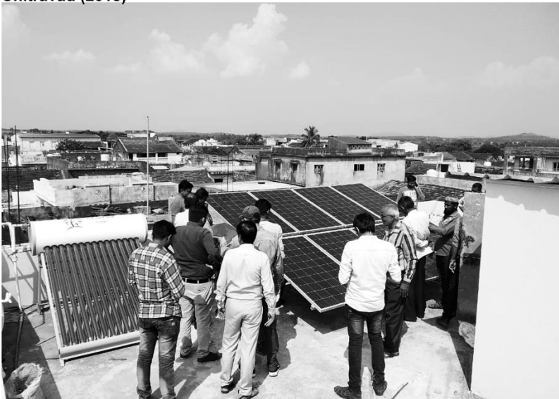
Fig 3.37 Harnessing clean energy - training masons on solar rooftop installations Chitravad (2018)
