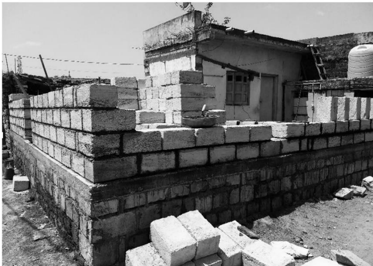
Fig 3.35 Use of locally available stones Optimization feature 2
