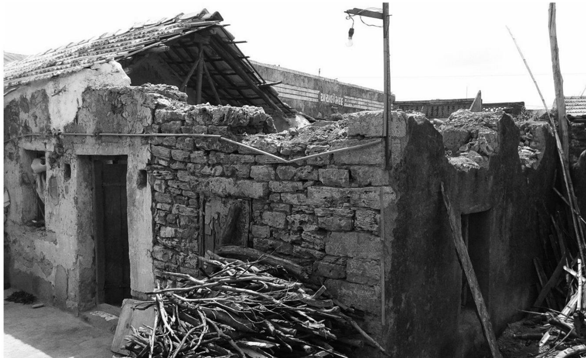
Fig 2.9 Dislodging of rubble and stones_Chitravad (2017)
