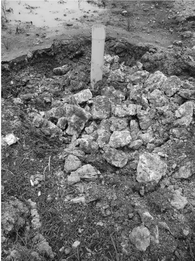
Fig 3.40 Soakpits with biofilters for grey water Chitravad (2019)
