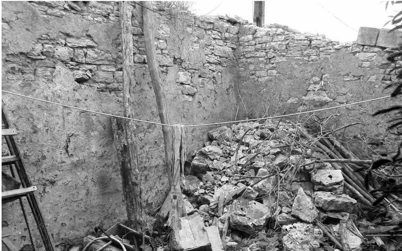
Fig 2.10 Dislodging of rubble and stones_Chitravad (2015)
