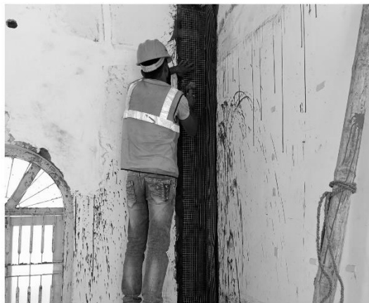
Fig 3.16 Using steel mesh for structural strengthening Chitrad (2019)
