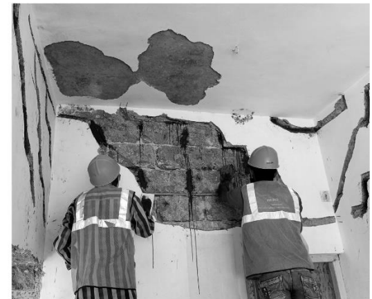
Fig 3.17 Treating the cracks before re-plastering Chitrad (2019)
