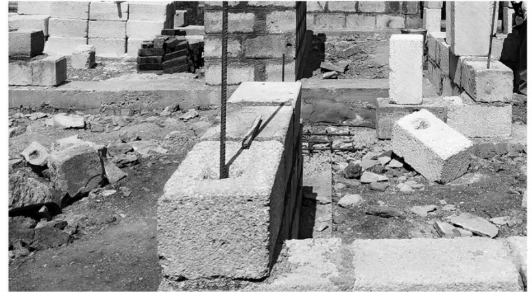
Fig 3.8 Corner reinforcement_Chitravad (2018)
