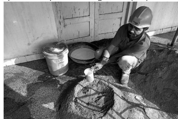
Fig 3.21 Mason making Polymer Modified Mortar_Chitradvad (2019)
