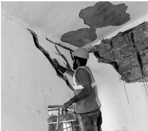
Fig 3.15 Sealing of crack Chitrad (2019)
