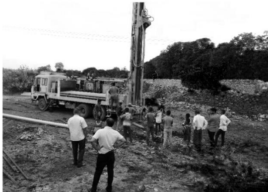
Fig 5.6 Recharge bore well drilling Chitradav (2019)
