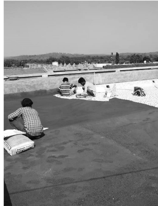
Fig 3.41 Cool Roof application Sangodra (2019)
