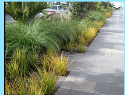
Figure 6 Image showing bioswale in Jellicoe Street, Auckland, New Zealand
