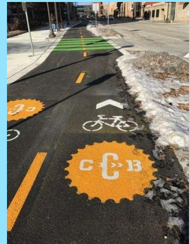
Figure 23 Image showing Permeable Pavements along Jackson street, St. Paul
