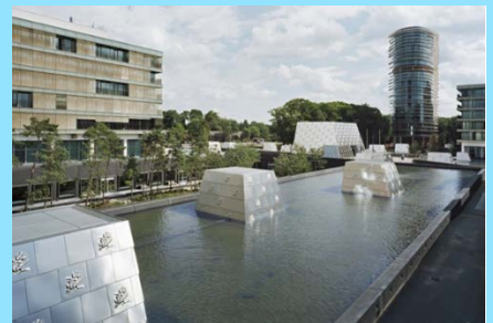
Figure 9 Image showing blue roofs in Walter Bos Complex, Apeldoorn
