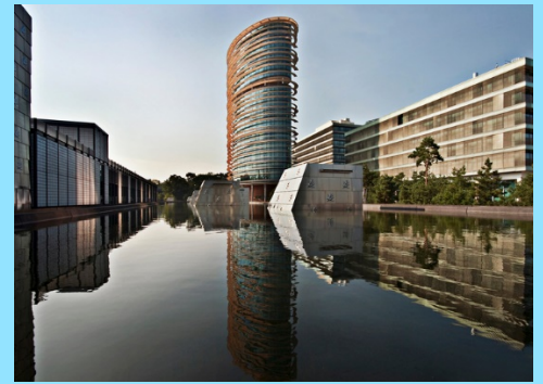
Figure 8 Image showing blue roofs in Walter Bos Complex, Apeldoorn
