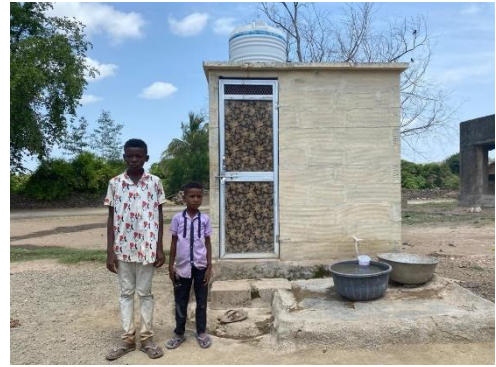
Figure 14. Sanitation unit constructed on site, Source: author
