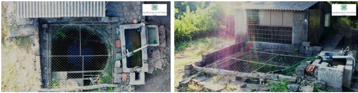
Figure 17. Well cover unit on site, source: author
