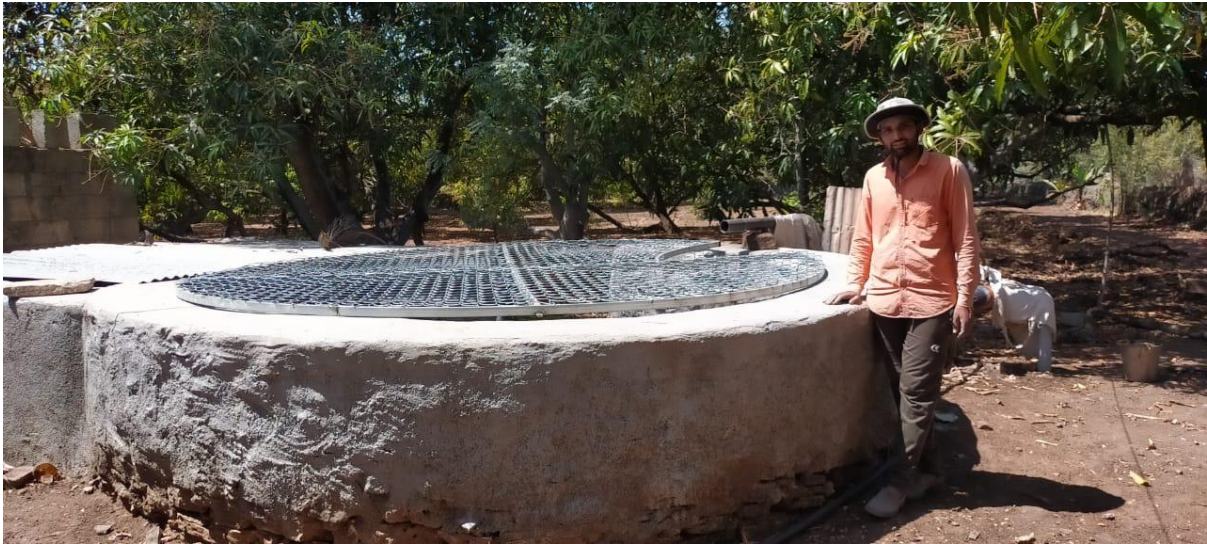
Covering of wells in the farmland in a project village carried out by AKAHI
