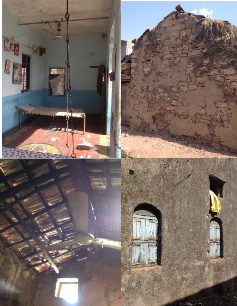
Figure 23 Flooring and interior wall finish, structure and external wall finish, wooden window shutter with opening options from 25 to 100%, roof structure and materials (Clockwise) (Source: Author)
