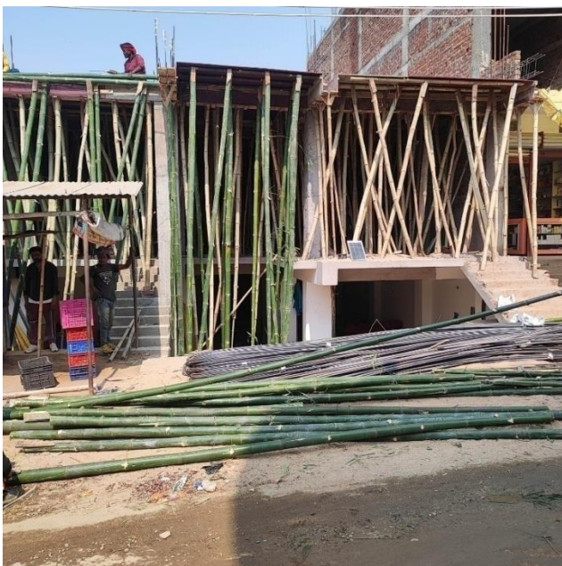
Bamboo Scaffolding for Construction
