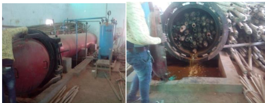
Bamboo Treatment in Pressure Vacuum Plant
