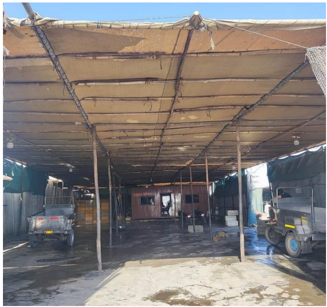
Bamboo Temporary Shop at Mangrol
