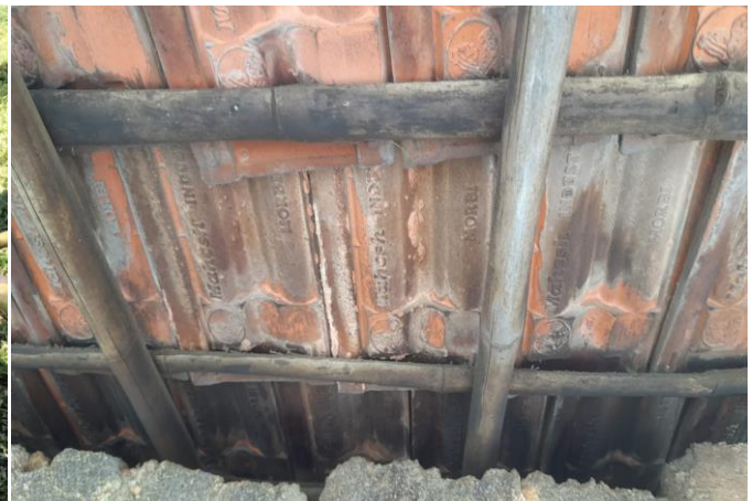
Bamboo Roofing after Smoke Treatment
